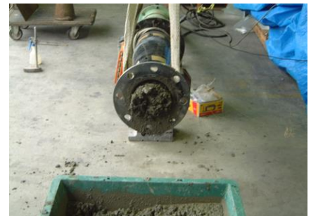
Continuous pumping without stopping
